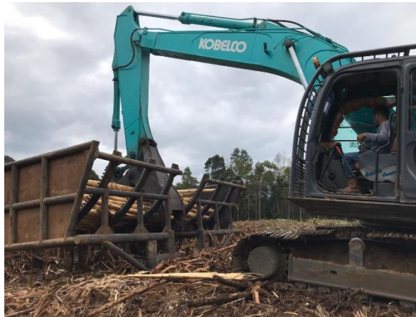
Jus Paku in Operation
