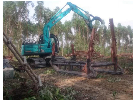
Poonton in Operation
